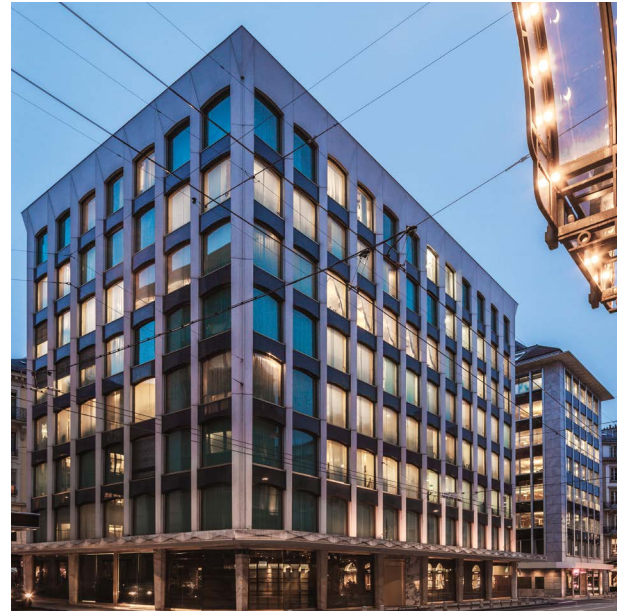
UBP headquarters at 96-98 rue du Rhône in Geneva
