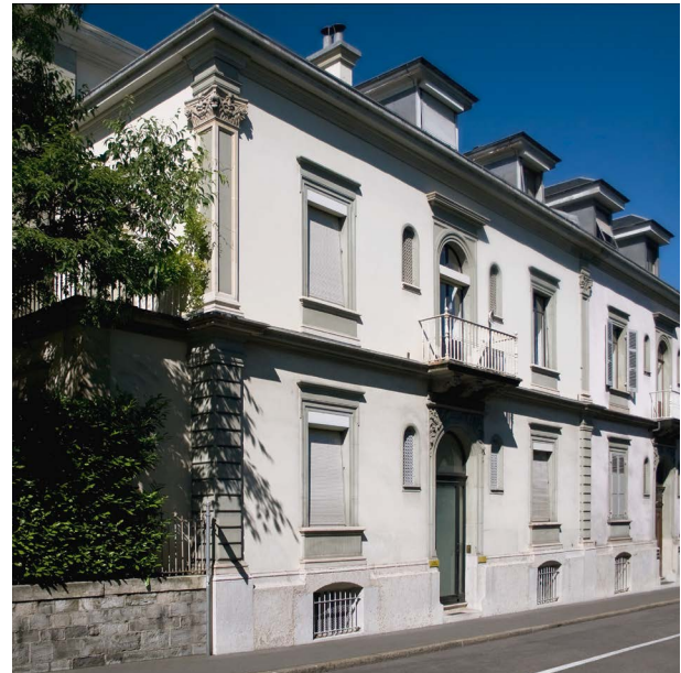
CBI's offices on the Cours des Bastions in Geneva from 1972
